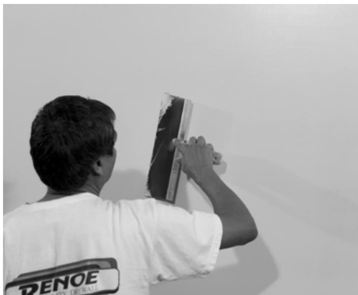
13. Compound buildup on the active surface of the speaker should not exceed 1/8" (3mm).
