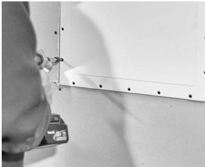
**TEST THE SPEAKER FOR 60 SECONDS WITH AN AUDIO SOURCE BEFORE COVERING WITH DRYWALL COMPOUND!**
