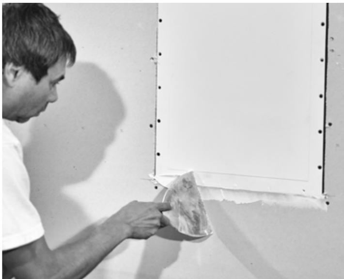
3. Allow hot mud to set slightly before applying mesh tape.
