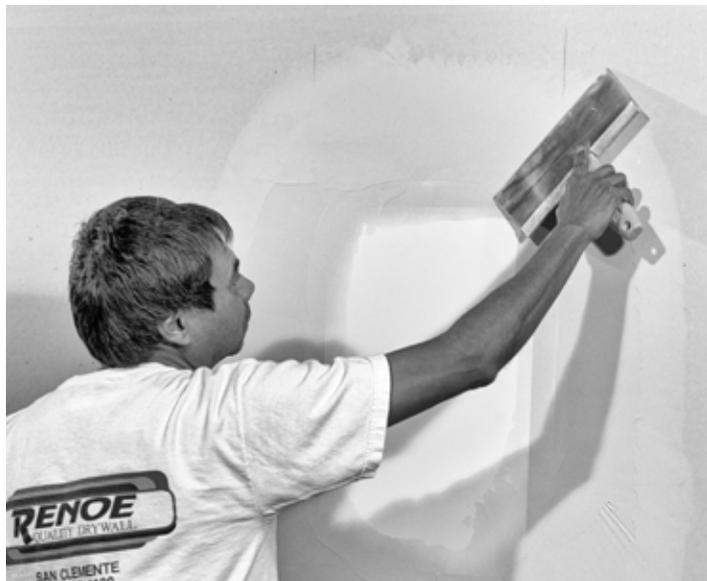
9. Build layers of compound as needed to obtain a flat surface.
