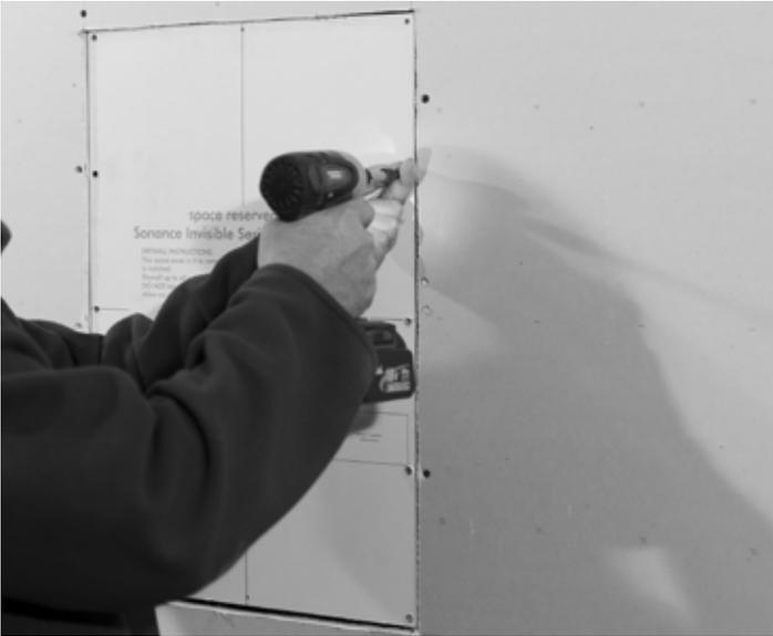
6. Be careful not to damage the exposed drywall during space saver removal.
