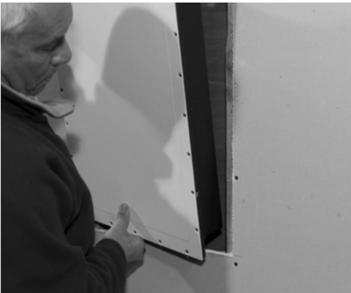
**13.** Secure speaker with at least 4 drywall screws on each side. Top and bottom are optional. Do not over tighten.
