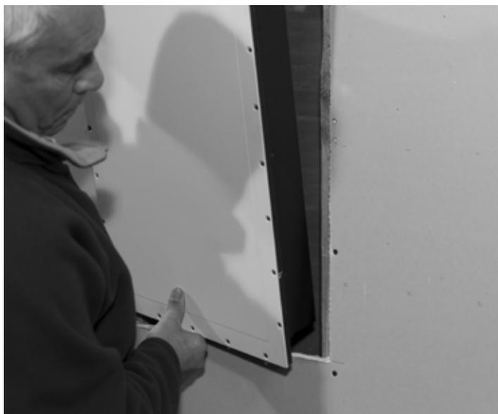
**15.** Secure speaker with at least 4 drywall screws on each side. Top and bottom is optional. Do not over tighten.
