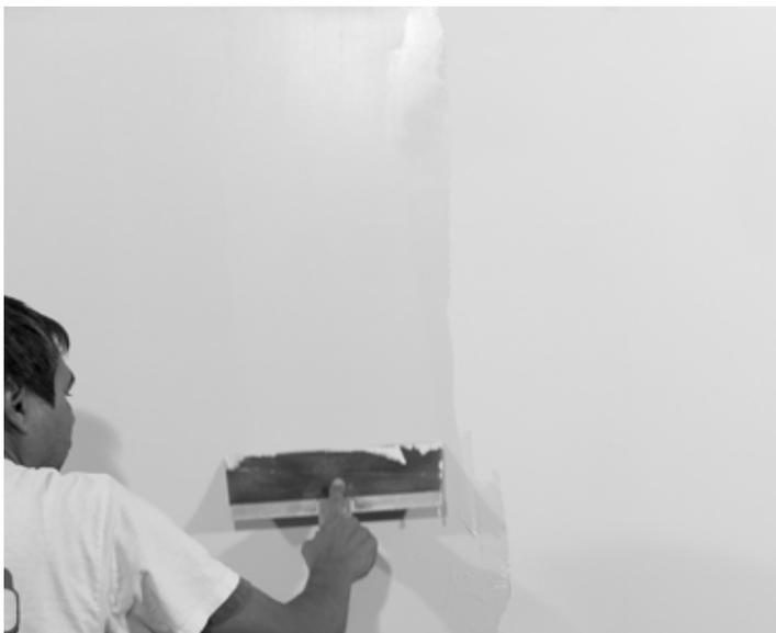
17. After final coat is applied and has dried, use a manual pole sander or block sander on entire wall (do not use a power sander). Wall surface should show no signs of a speaker. If any defect is found, skim coat entire area, and sand down again.
