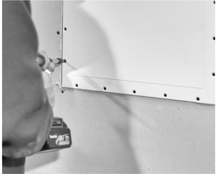
**TEST THE SPEAKER FOR 60 SECONDS WITH AN AUDIO SOURCE BEFORE COVERING WITH DRYWALL COMPOUND!**
