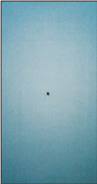
Drill a small exploratory hole
