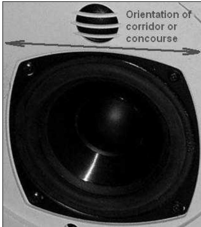
**2-way ceiling loudspeaker orientation**
