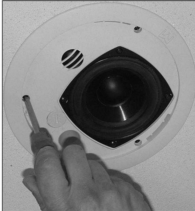
**Tightening the swivel-tab screws**
